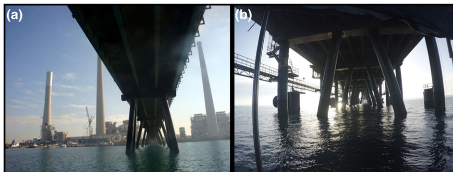
FIGURE 2 Hadera infrastructure site: Orot Rabin Power Station coal conveyor and jetty infrastructure above water and under the conveyor. (a) Coal conveyor piles. (b) Coal jetty piles
