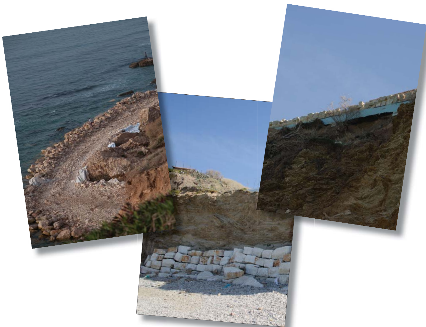
Measures taken to protect a Crusader castle (Appolonia - left) from erosion and protections taken by private property owners (Bet Yanai - center and right) in Israel.
