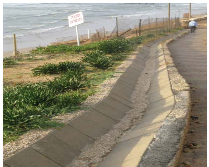
Drainage to prevent erosion in Herzliya, Israel.
