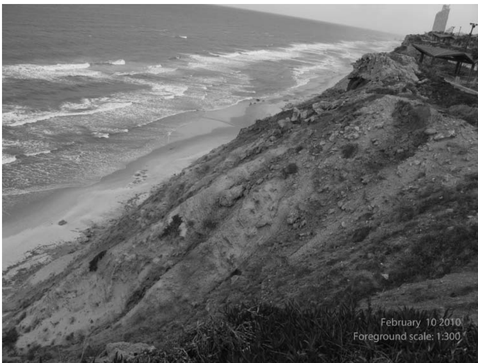
Figure 2. Northward view of the eroding coast over Segment J (highest erosion) and Segment H (high erosion) with recreational structures in the distance. Cliff height \sim 30 m.
